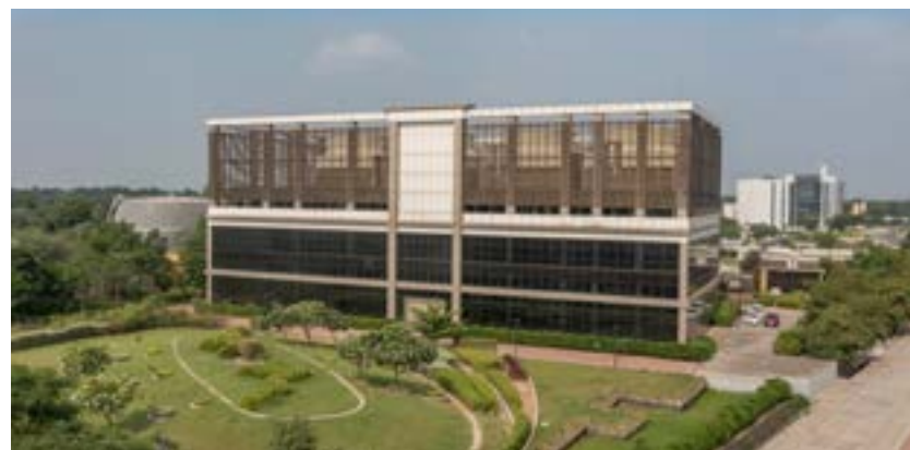
INDIA'S FIRST DISTRICT COOLING SYSTEM
